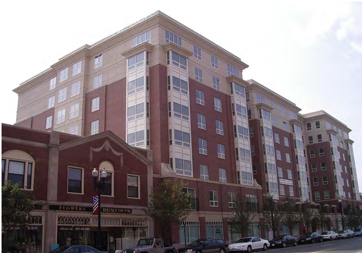
While too tall to meet the Marlborough height limits, this shows a very successful addition on top of an existing structure. The articulated front helps to break the massing of the apartments above the first floor retail. Compatible materials are used.
