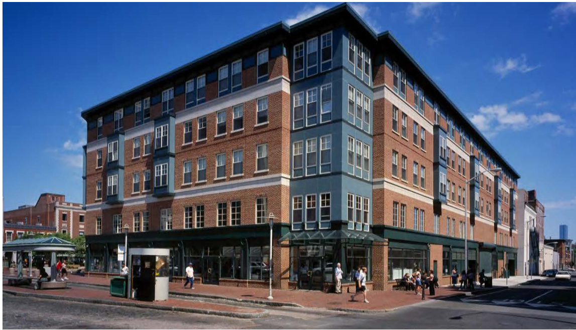
An example of a corner building with active retail on both street frontages.
