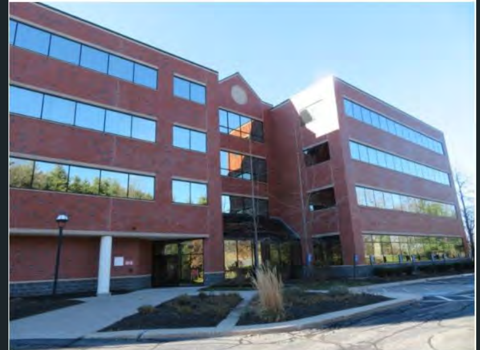
Physik Instrumente plans to move to this building on Lizotte Drive, should the city approve a TIF agreement. (Photo/Maureen Sullivan)
